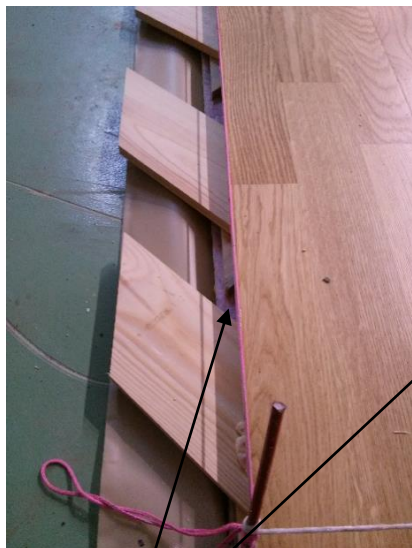
Before the top flooring is installed please use the chalk line to set the correct position of the flooring (straightness).
