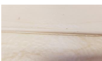
The presence of a small bump indicates the perfect level of fusion of the welding rod.
